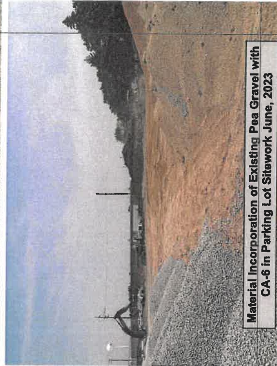
Backfilling Old MacArthur Basement June, 2023
